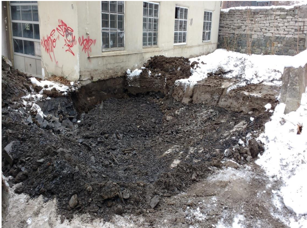
Photo 7 - Surexcavation de EX-3.
